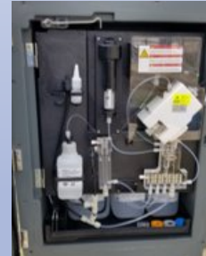
Amtax sampler measuring ammonium
